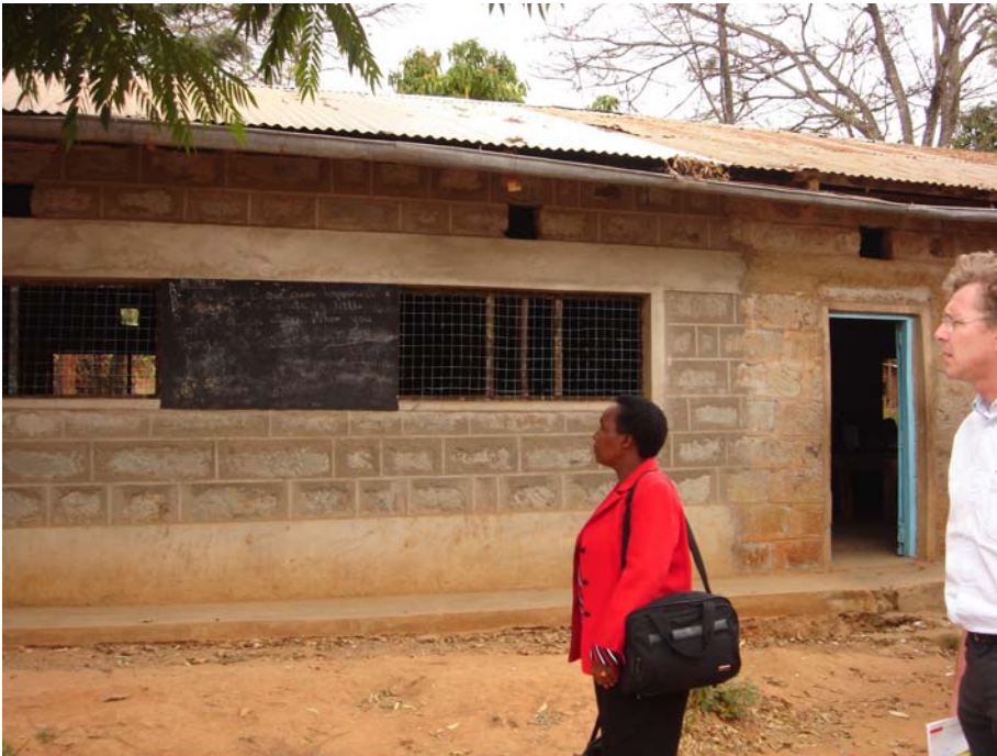
New Classrooms constructed in Mbeere District Kenya with funding from CDF
