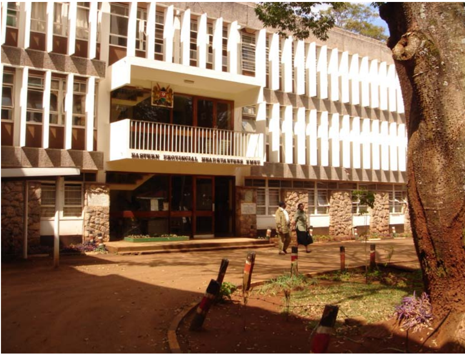
Provincial Headquarters of Eastern Province in Embu Town – its architecture a reflection of its past substantive status – significantly imposing compared to LA or CDF offices.
