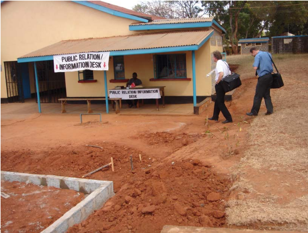
Office of the Local Authority in Mbeera – with recently established “Public Relations Desk” on the veranda
